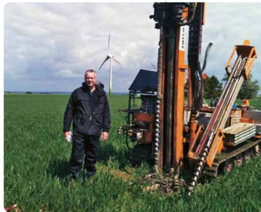
Thomas Hansson overseeing sample drilling at the ESS site.
